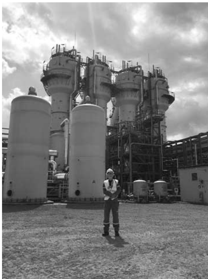
The author at the Steelanol waste-gases-to-ethanol facility, Ghent, Belgium, 6 June 2024.
